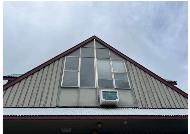
Figure 4 Window - northern end. Note the deterioration of both window and cladding fabric. Source: Kosciuszko Thredbo Pty Ltd, 18.05.23
