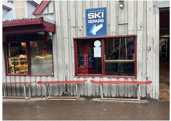
Figure 2 Facing Avalanche cafe. Note cladding deterioration. Source: Kosciuszko Thredbo Pty Ltd, 18.05.23
