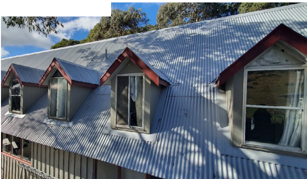
Figure 5 Staff accommodation windows, north elevation. Note deterioration of the roofing, poor condition of and installation of inappropriate sliding windows and some deterioration of timber cladding. Source: Statement of Environmental Effect for Valley terminal building Thredbo NSW, Accent Town Planning Pty Ltd, February 2023
